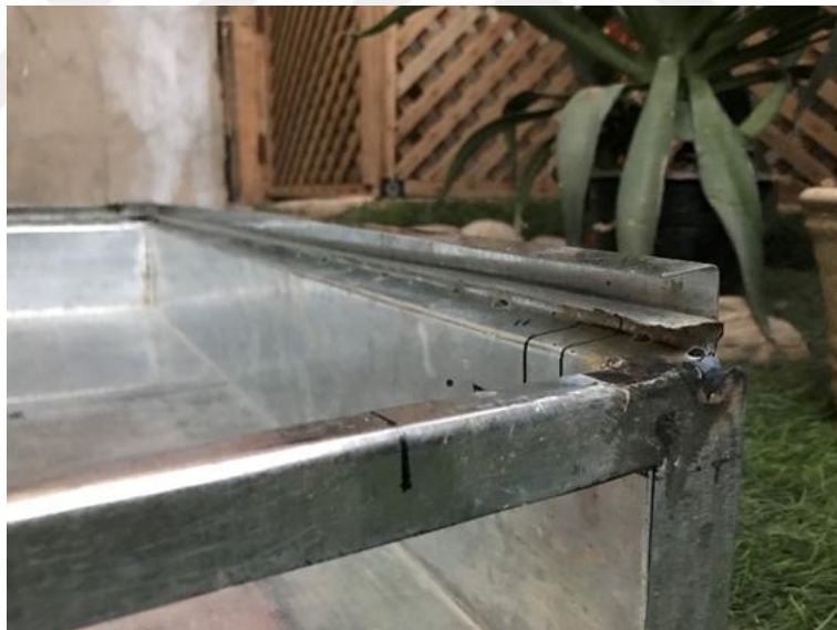
Figure 3.4: Close view of the position of the glass in the enclosure.
