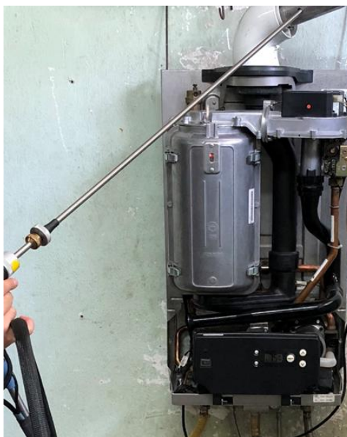
Figure 5. Measuring pollutant gas emissions by ECOM J2KN analyzer
