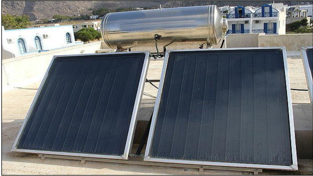
Figure (2.3): typical flat-plate collector.
